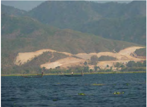
Hotel Zone landscaping works from Inlay Lake
