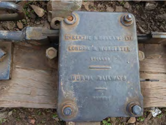
Original infrastructure from Burma Railways
